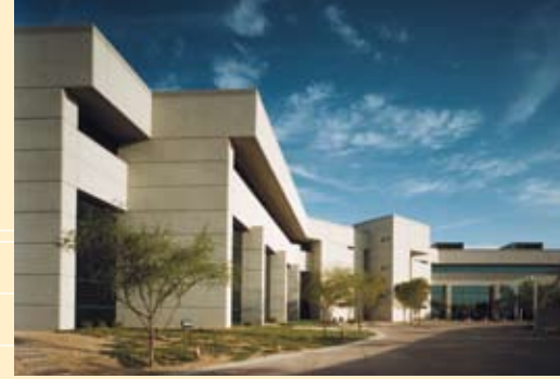
Fig. 9 – Cantilevered floor used to shade windows.
