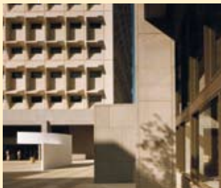
Fig. 11 – Deep recessed windows and overhang (eggcrate device). Photo: © MBA
