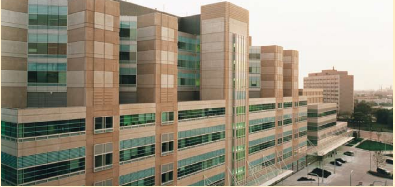
Fig. 36 – Insulated sandwich wall panels. John H. Stroger, Jr. Hospital of Cook County, Chicago, IL CCH Design Group headed by Loebl Schlossman & Hackl Photo: @Hedrich Blessing
