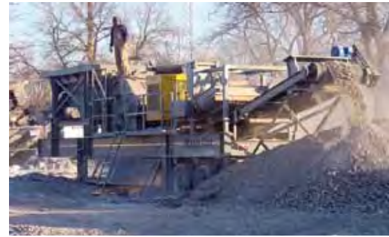
Figure 9 Crushed concrete from other sources can serve as recycled aggregate.
