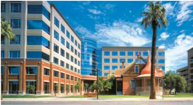
Figure 4(a) Arizona Department of Administration (ADOA), Phoenix, Ariz. Architect: Opus Architects and Engineers
