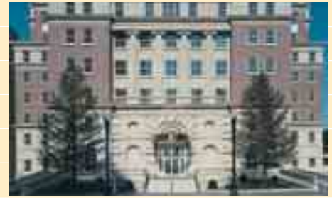
Fig. 4: Color and detailing of the precast members at the Peachtree Office Condominium were developed to complement adjacent historical structures constructed of brick and limestone.
