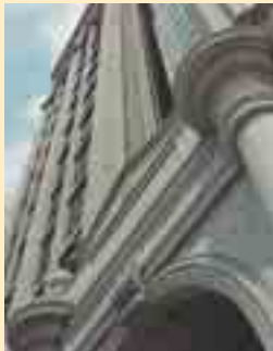
Fig. 1: At the Jefferson Pilot Corporate Headquarters addition in Greensboro, N.C., sandblasted precast panels were used in the design of the new structure to reflect the scale and character of the terra cotta cladding of the original building.
