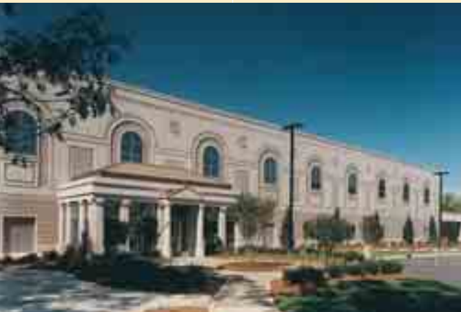
Fig. 7: Designed to withstand extreme wind and seismic loads without resembling a bunker, this data-processing center uses load-bearing precast concrete wall panels and structural precast floor and roof slabs.
