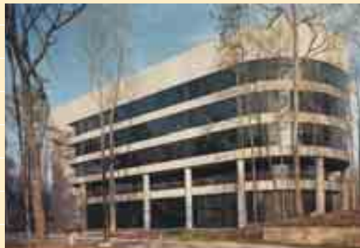
Fig. 5: The Chick-fil-A corporate headquarters in Atlanta has added an annex, constructed 15 years after the original, that is clad with the same precast mix design and panel detailing, seamlessly blending the two structures into a corporate campus.
