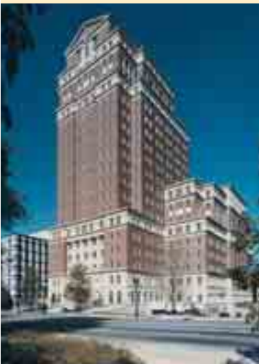
Fig. 3: Buff-colored precast was used for cornices, trim members, sills and belt courses in conjunction with hand set brick to compose the classically proportioned façade of the Peachtree Office Condominium in Atlanta.
