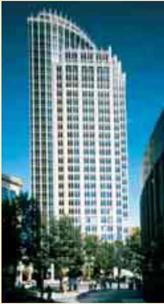
Fig. 6: The IJL Corporate Headquarters in downtown Charlotte, N.C., features two colors of sandblasted precast concrete along with granite clad precast panels.
