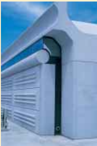
The use of the bullnose sections on various support buildings at the Hyperion Wastewater Treatment Facility broke up the flat-panel facade and created a distinctive look.
