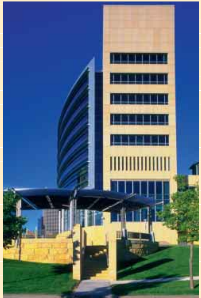
Precast cladding blended with the stone base of the Federal Reserve Bank in Minneapolis, Minn.
