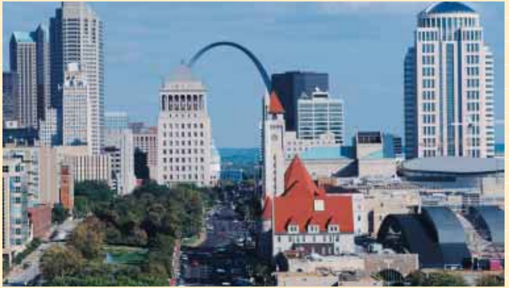
The multi-color precast exterior of the 29-story Thomas F. Eagleton United States Courthouse, St. Louis, Mo., stands out as one of the most unique skyscraper dotting the skyline.
